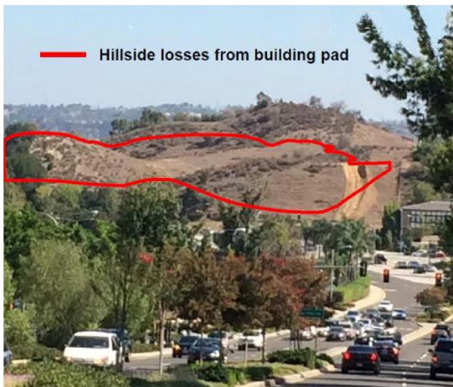
Hillside Losses from Dirt Building Pad with Asphalt Cover visible from Grand Avenue Entering
